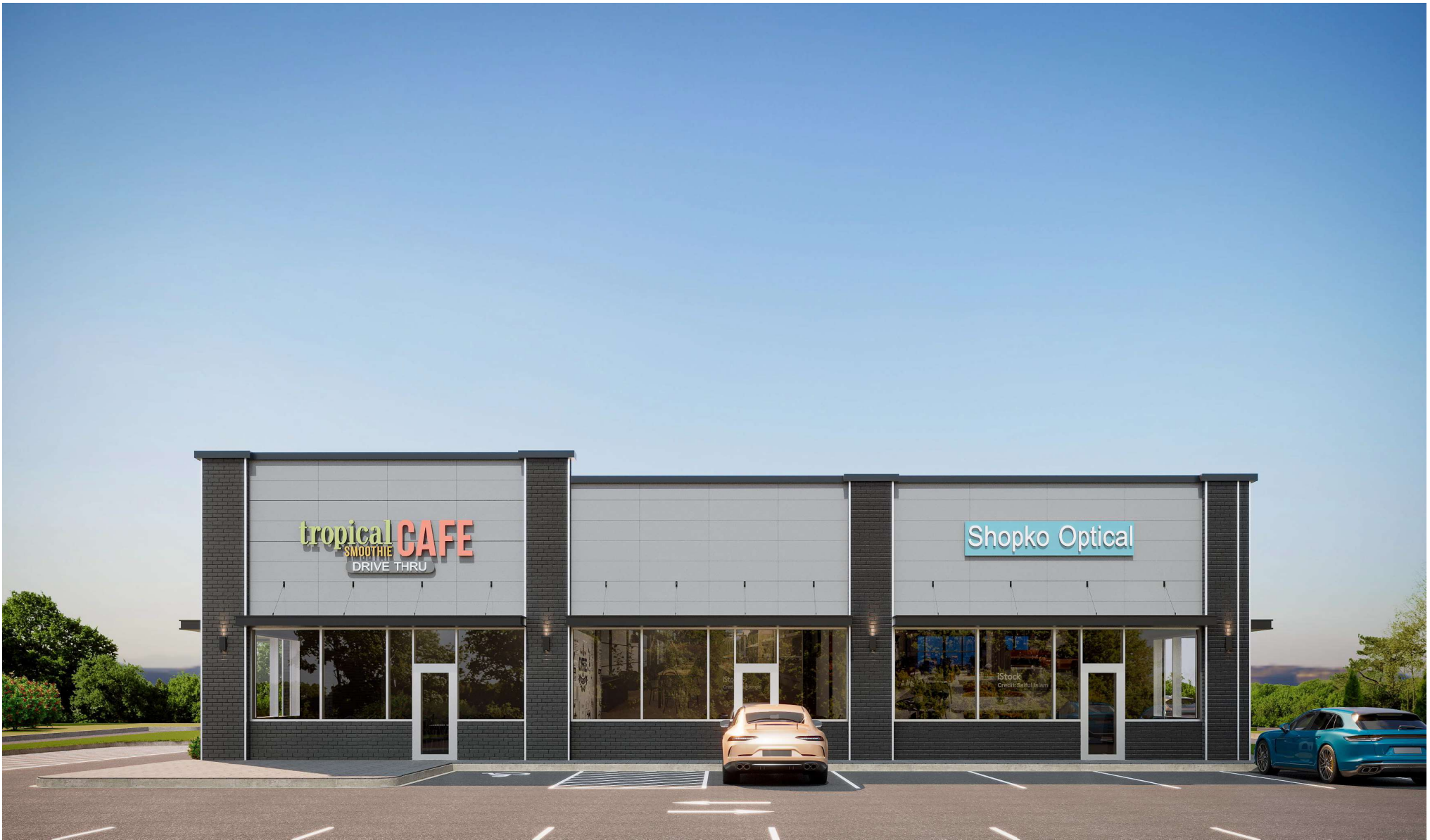
EXTERIOR NORTH SIDE - MARKET CENTRE
