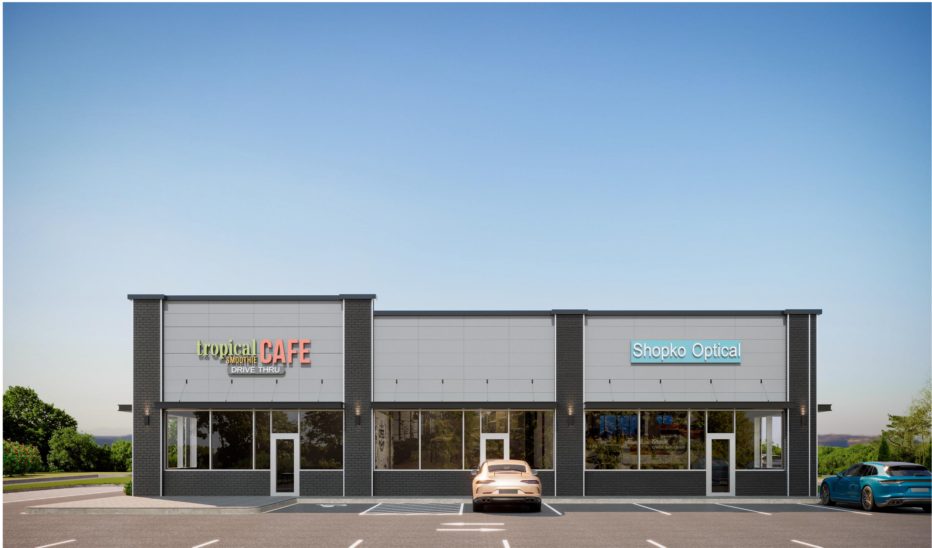
EXTERIOR NORTH SIDE - MARKET CENTRE
