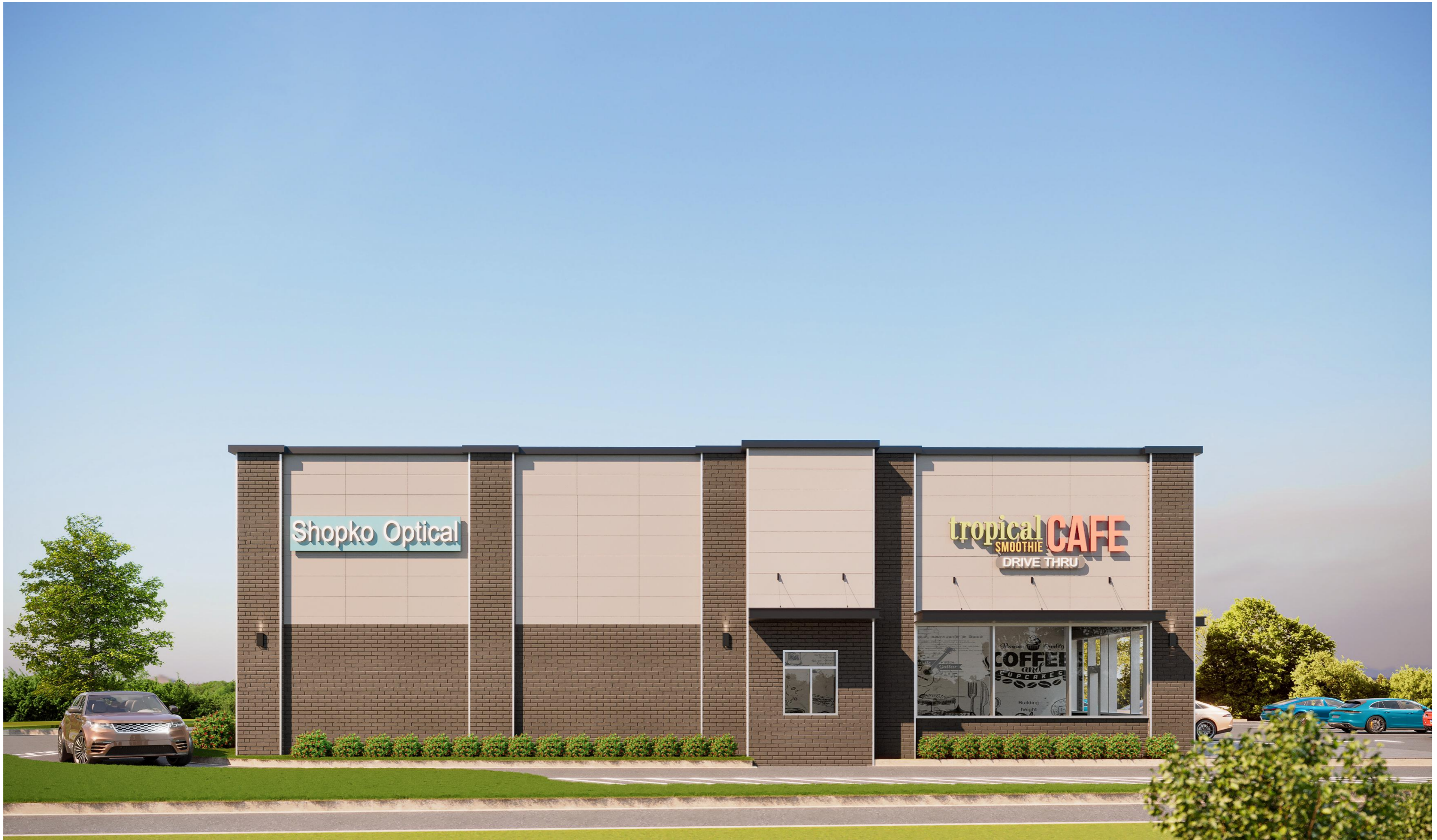
EXTERIOR EAST SIDE- MARKET CENTRE
