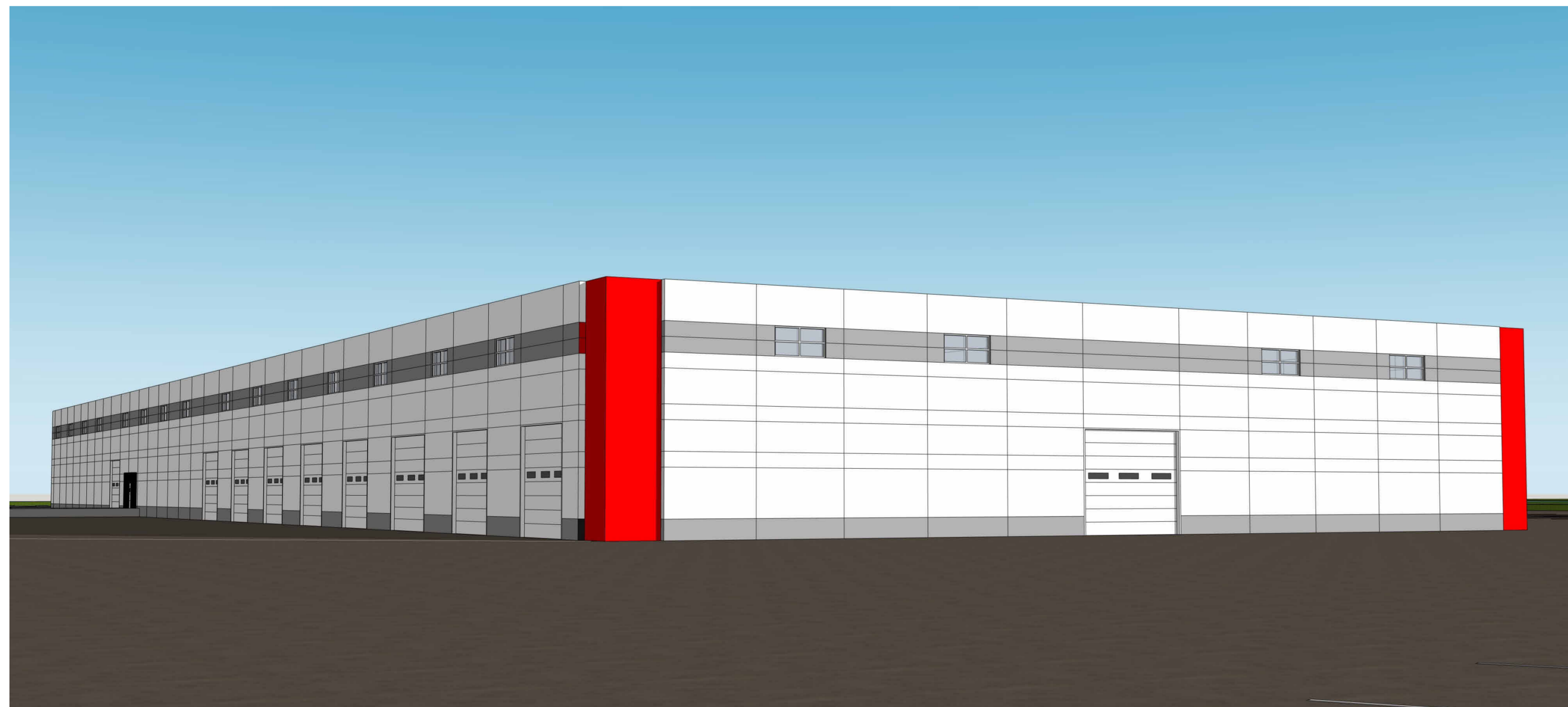
VIEW FROM NORTH WEST CORNER
