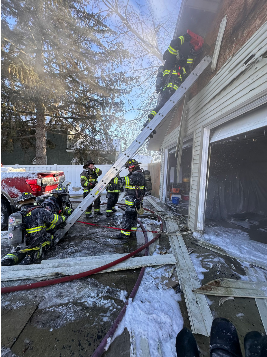
January 16 th , crews battled a garage fire on Hwy E in extreme cold weather conditions. Wind Chills were below zero. Several of the Somers personnel on scene had just returned from helping fight building fires in the Village of Salem Lakes overnight. Equipment and clothing were frozen solid.
