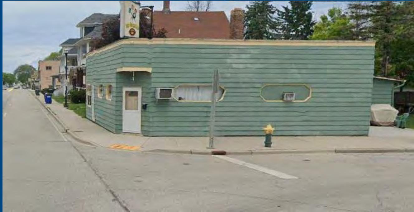
NW quadrant of WIS 32/23 rd St.
