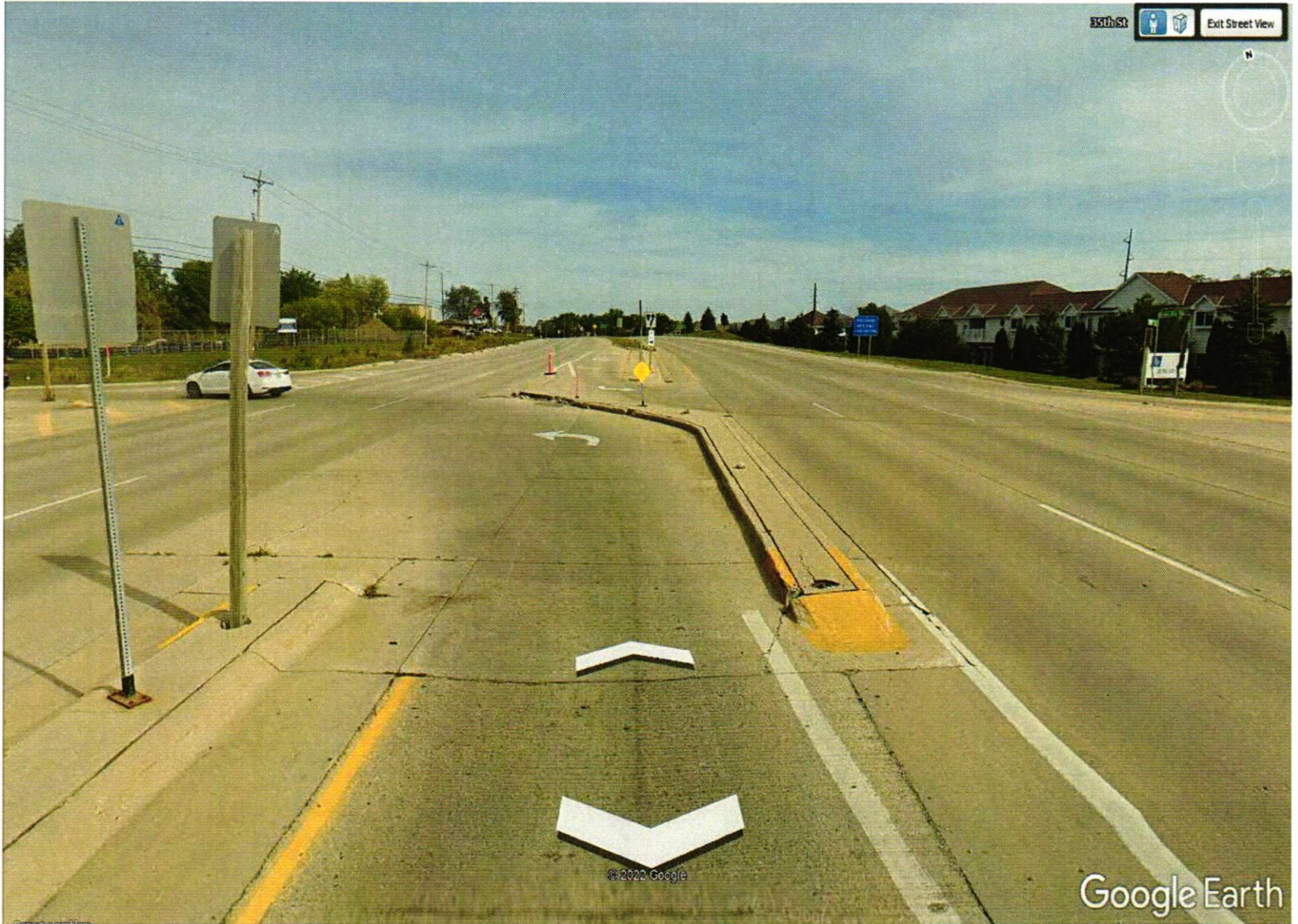
NB STH 31 (looking North approaching intersection)
