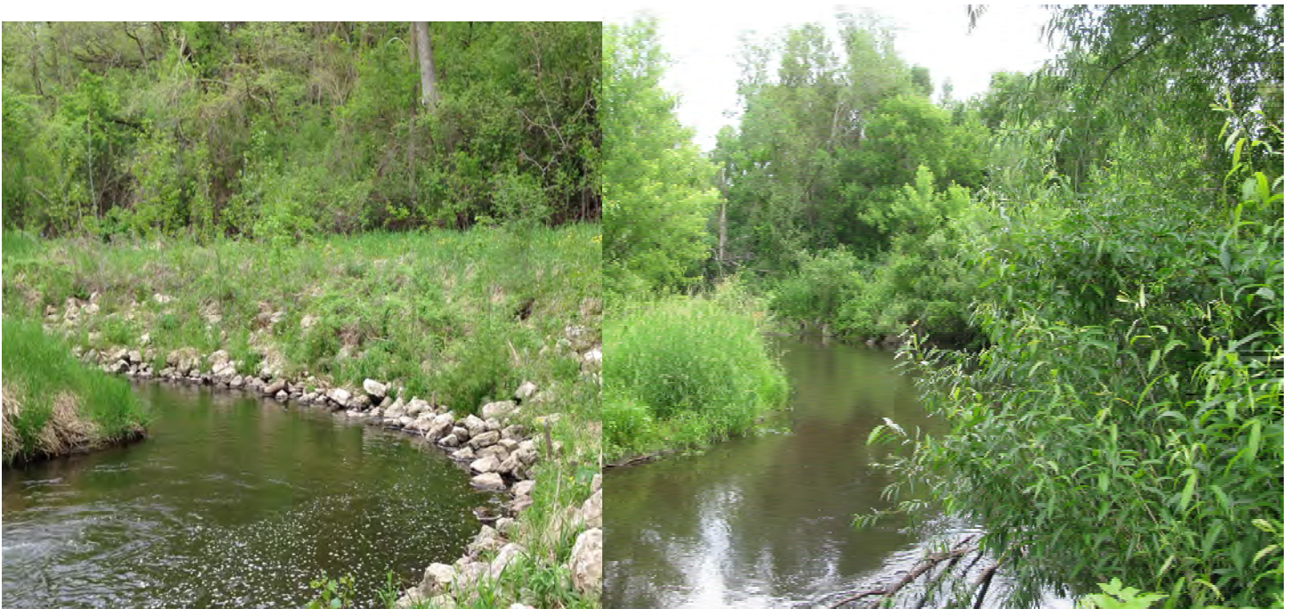
Figure 7. Left—A constructed stone toe and bioengineered bank after 2 years of growth. Right—A constructed stone toe and bioengineered upper bank after 10 years of growth. Neither bank requires long term maintenance.
