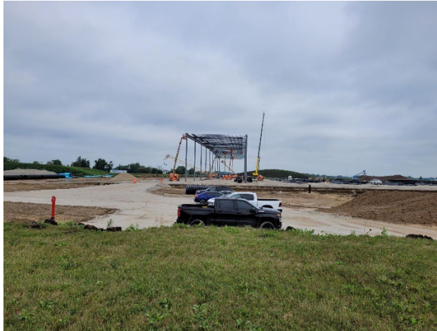
First Park 94 Building “D”
