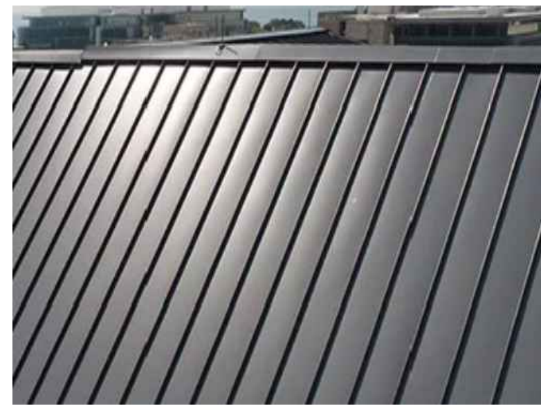
PROPOSED ROOFING FAC-CLAD: SNAP-CLAD STANDING SEAM ROOFING WITH 12" O.C. RIBS, DARK GRAY COLOR
